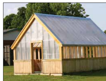
The greenhouse nearing completion.
